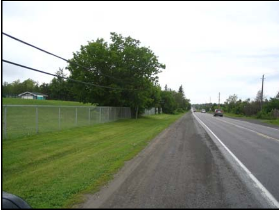
Plate 9: View to southeast along Carp Road near main entrance to WM facility. Disturbed ROW and adjacent lands.
