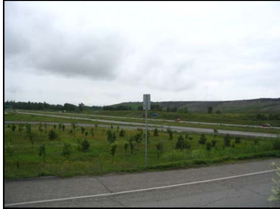
Plate 10: View to west across Hwy 417 from Carp Road. Note berm along southeast edge of existing facility and landfill hill.
