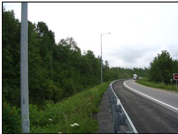
Plate 12: View to east along ramp from Hwy 417. Adjacent ditch and lands are disturbed and wet.
